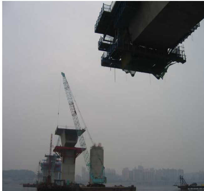
Figure 15. Construction of FCM bridge.
